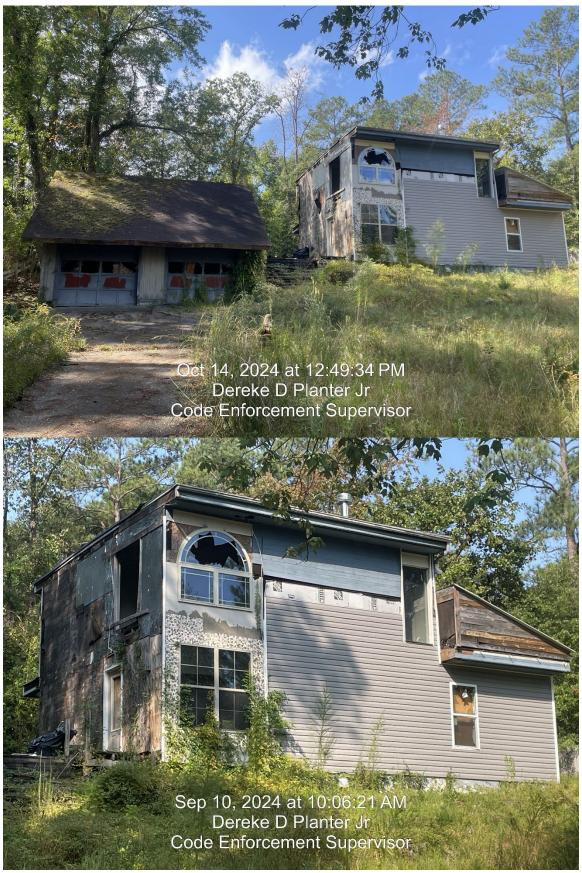
(Roof covering shall not be loose, nor have holes or leaks; No rafters shall be rotted, broken, sagging excessively; All exterior finish shall be weathertight without excessive holes, cracks or rotted boards which permit air or water to penetrate rooms)
