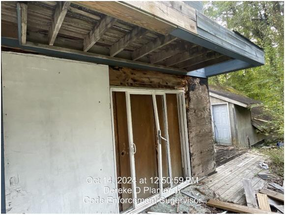
(All finish shall be weathertight without excessive holes, cracks or rotted boards which permit air or water to penetrate rooms; roof covering shall not be loose, nor have holes or leaks; Windows shall be reasonably weathertight with no broken glass)
