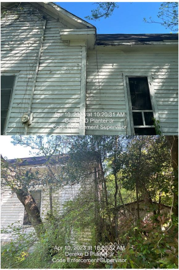
(Roof covering shall not be loose, nor have holes or leaks; ll exterior finish shall be weathertight without excessive holes, cracks or rotted boards which permit air or water to penetrate rooms)
