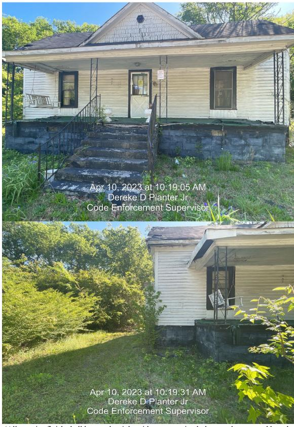
(All exterior finish shall be weathertight without excessive holes, cracks or rotted boards which permit air or water to penetrate rooms; Stairs and steps shall be free of holes, grooves and cracks large enough to constitute accident hazards; Every porch which is more than three feet high shall have rails not less than 30 inches above the floor.)
