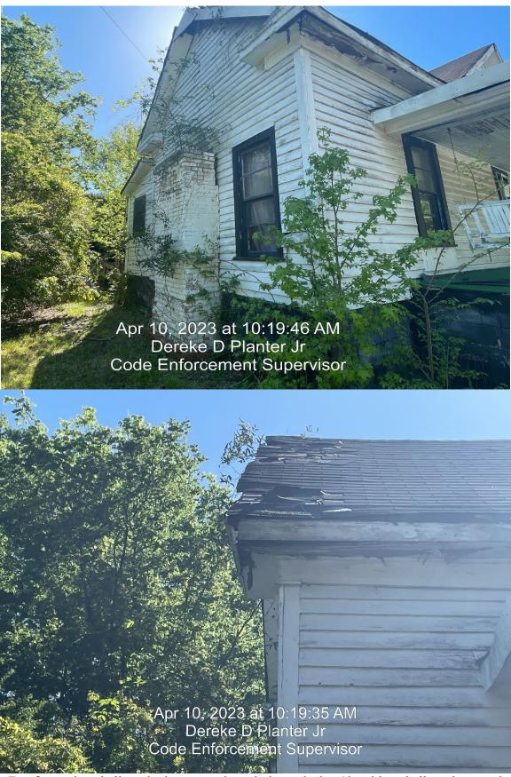
(Roof covering shall not be loose, nor have holes or leaks; Sheathing shall not be rotted, loose or sagging excessively)
