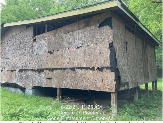
(Piers shall be sound; footings shall be sound with adequate bearing)
