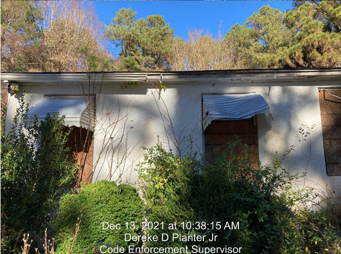
(exterior finish not weathertight, Roof covering loose, with holes or leaks.)
