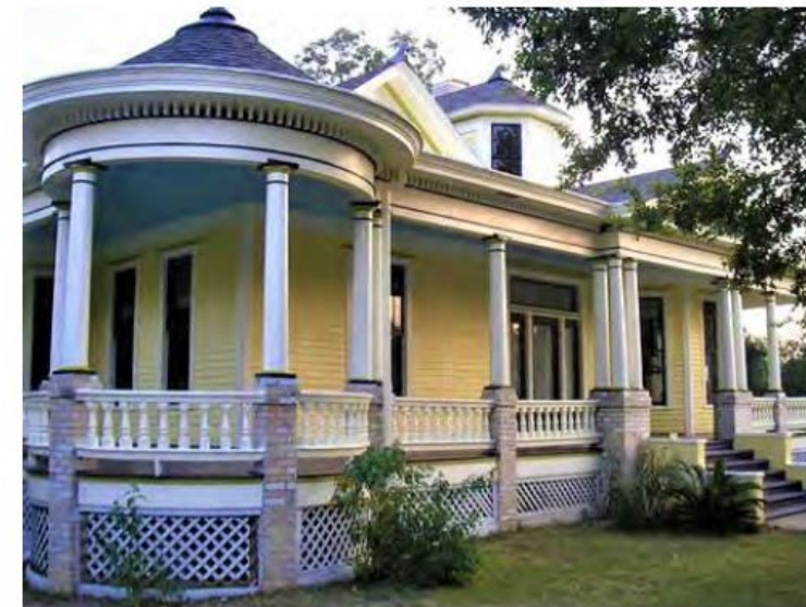
The above example shows how lattice work can be used as screening between brick piers at the foundation.
