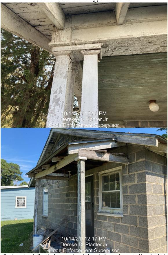
(Roof covering shall not be loose, nor have holes or leaks; cracks or rotted boards which permit air or water to penetrate rooms; adequate posts and railings, not rotted, broken or termite damaged, shall be provided)
