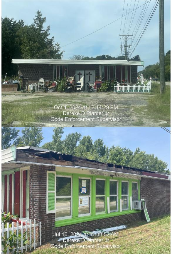
(No rafters shall be rotted, broken, sagging excessively; All exterior finish shall be weathertight without excessive holes, cracks or rotted boards which permit air or water to penetrate rooms)
