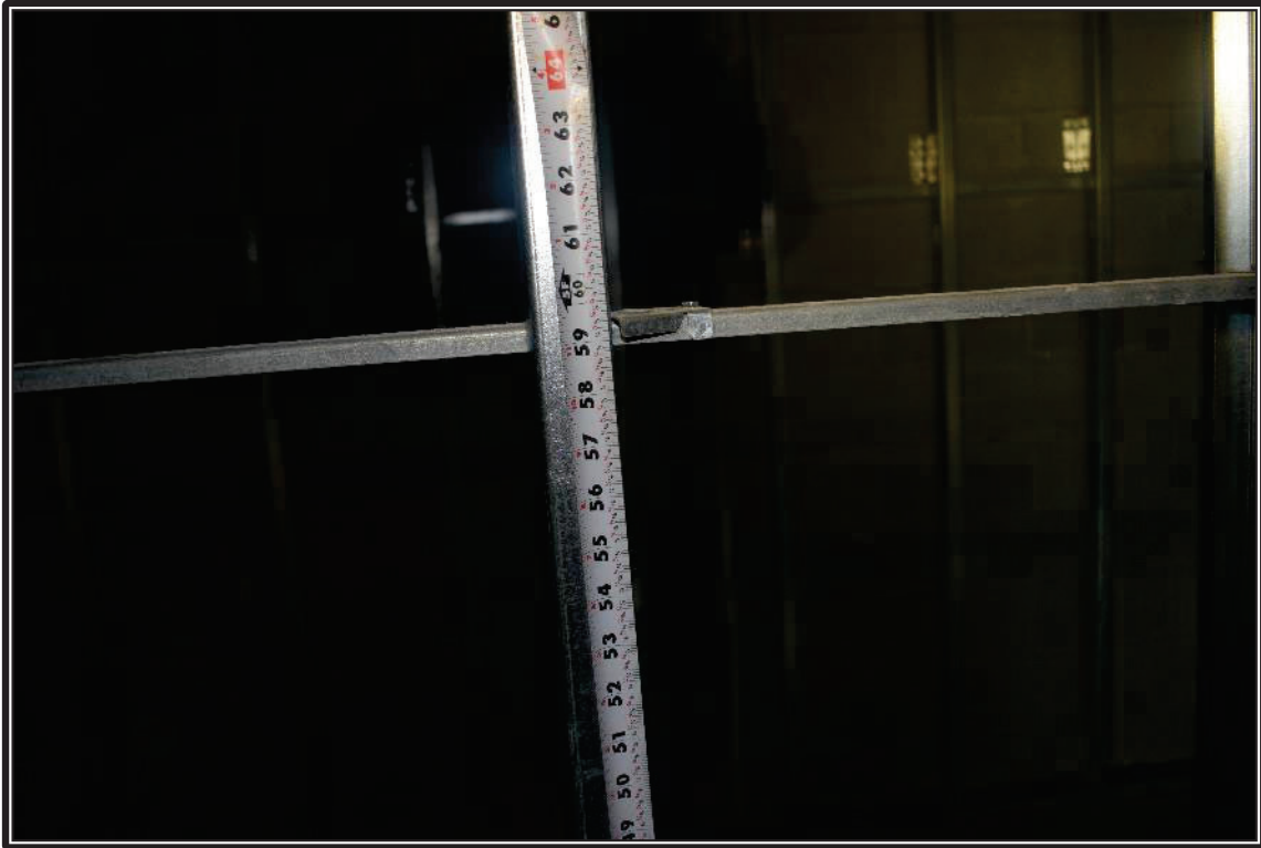
Photo 13: Representative view of the measured distance to the first row of bridging above the concrete slab.
