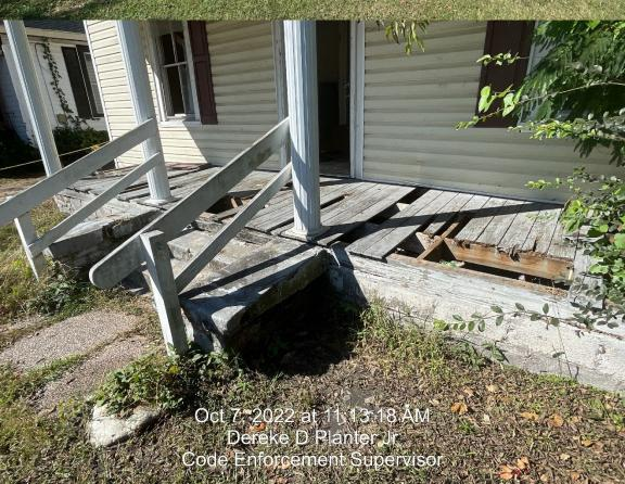
(Adequate posts and railings, not rotted, broken or termite damaged, Roof covering shall not be loose, nor have holes or leaks)
