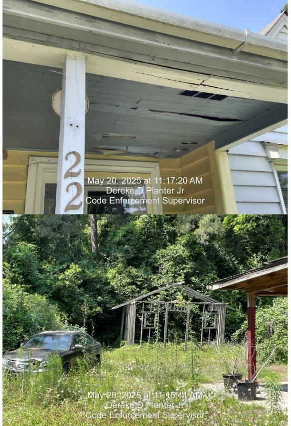
(Wall finish shall be free of holes and excessive cracks which permit air to penetrate rooms, Adequate posts and railings, not rotted, broken or termite damaged, shall be provided. )
