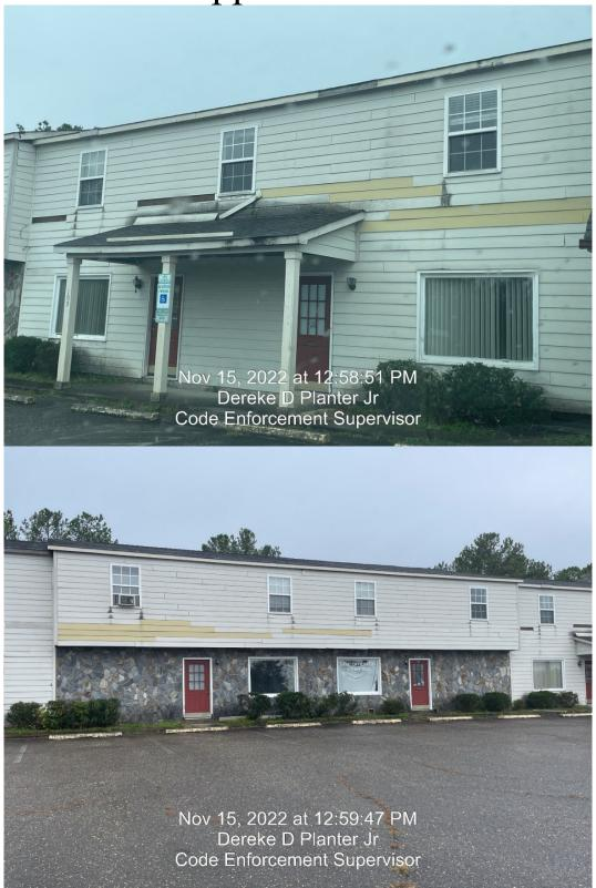
(Exterior walls with excessive holes, cracks and rotted boards which permit air or water to penetrate)
