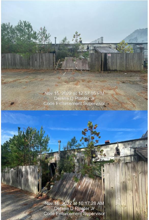
(Exterior walls not weathertight with excessive holes, cracks and rotted boards which permit air or water to penetrate rooms.)
