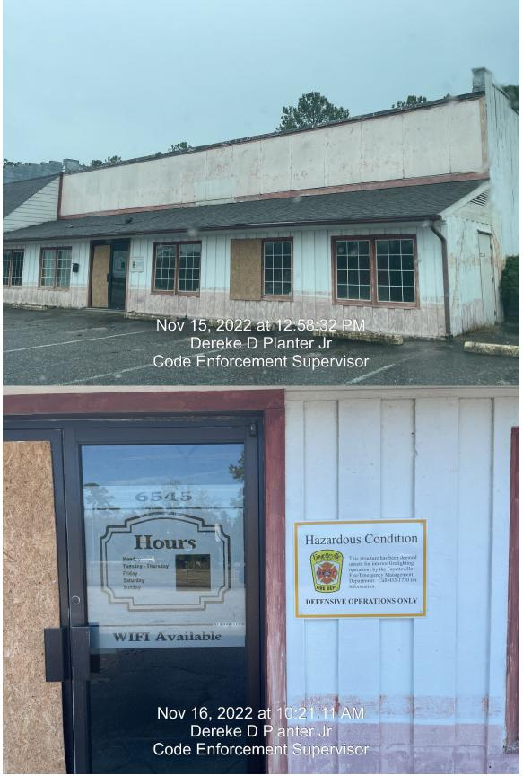
(Roof coverings to be be rotted, loose or sagging excessively. Structure was deem unsafe for interior firefighting operations.)
