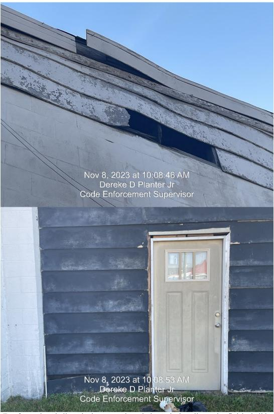
(Roof covering shall not be loose, nor have holes or leaks; all exterior finish shall be weathertight without excessive holes, cracks or rotted boards which permit air or water to penetrate rooms;)
