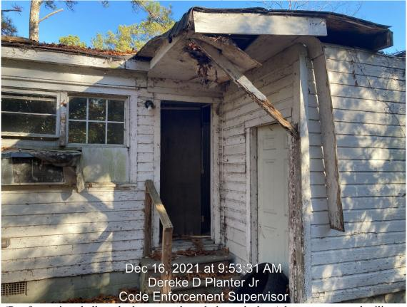
(Roof covering shall not be loose, nor have holes or leaks; Adequate posts and railings, not rotted, broken or termite damaged, shall be provided; Steps supports shall not be rotting, sagging or deteriorating)
