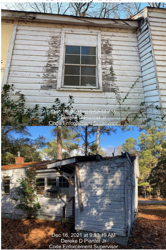
(All exterior finish shall be weathertight without excessive holes, cracks or rotted boards, not rotted, broken or termite damaged, shall be provided; Roof covering shall not be loose, nor have holes or leaks)
