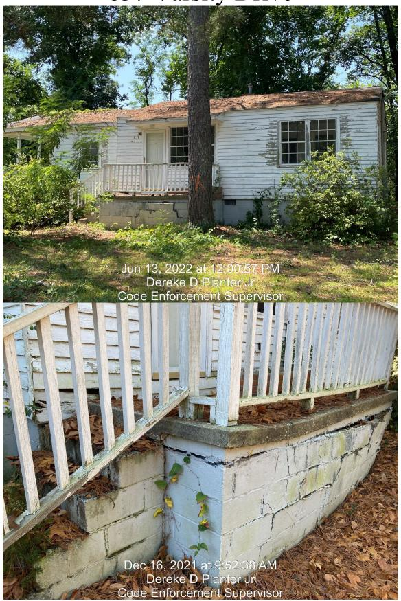
(Foundation not firm ground; water shall be permitted to stand under such dwelling or structure. Il exterior finish shall be weathertight without excessive holes, cracks or rotted boards which permit air or water to penetrate rooms)
