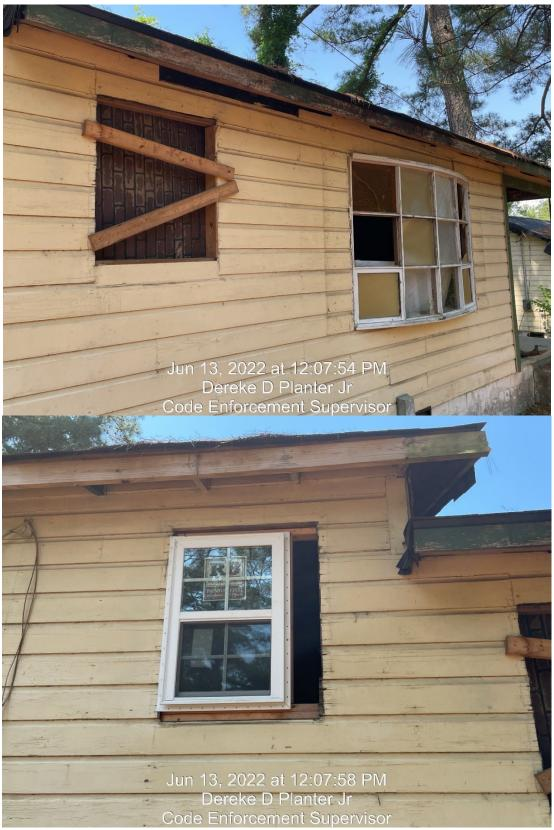
(All exterior finish shall be weathertight without excessive holes, cracks or rotted boards which permit air or water to penetrate rooms; Roof covering shall not be loose, nor have holes or leaks; Windows shall be reasonably weathertight with no broken glass)
