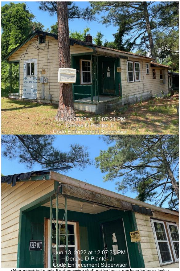
(Non-permitted work; Roof covering shall not be loose, nor have holes or leaks; improperly supported ends)
