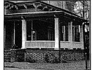
The brick pier foundation of the Mansard Roof House has been infilled with lattice-patterned brick. The walls retain the original wood siding and decorative details.
