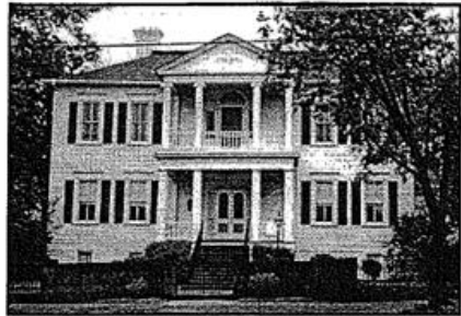
The wood-frame Sandford house is built on a raised brick basement.
