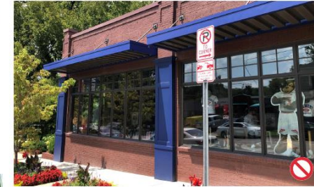
While attractive, these added wooden pilasters create a false sense of history.
