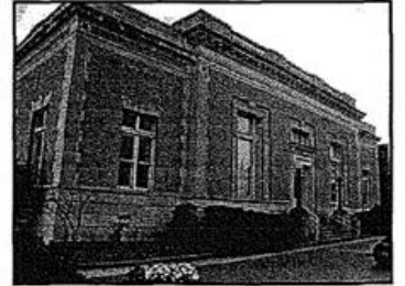
The (former) U.S. Post Office on Hay Street is built on a stone foundation. The brick walls are accented by stonequoins and cornices.
