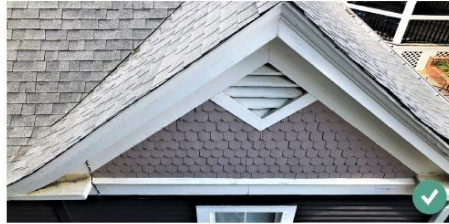
This vent and wood fishscale shingles have been well preserved.
