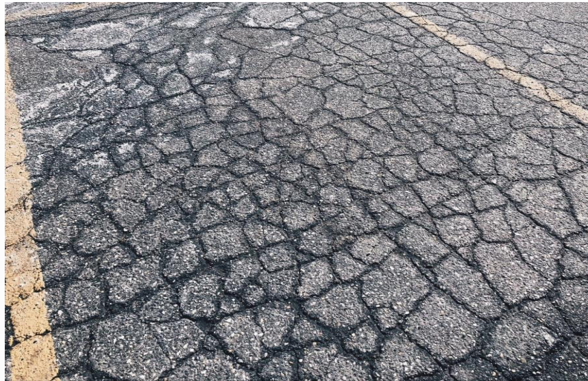
Alligator Cracking
