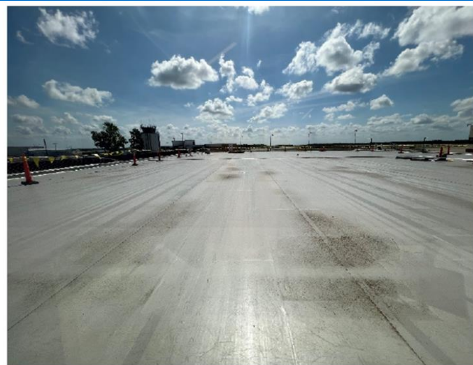
Baggage Claim roofing installation
