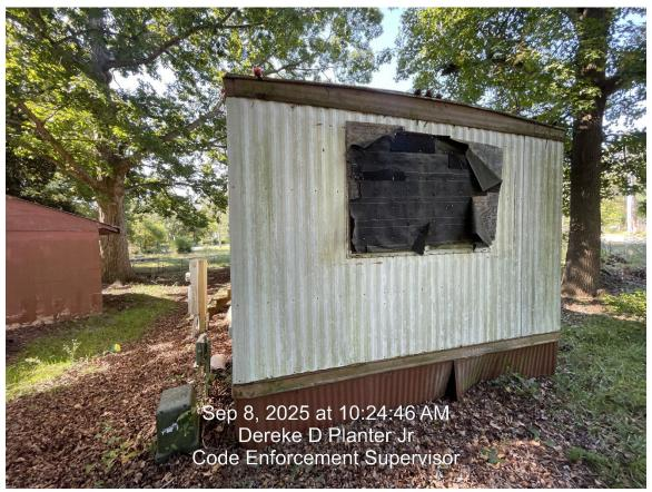
(All exterior finish shall be weathertight without excessive holes, cracks or rotted boards which permit air or water to penetrate rooms;)
