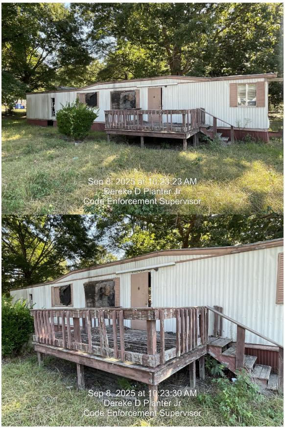
(All exterior finish shall be weathertight without excessive holes, cracks or rotted boards which permit air or water to penetrate rooms. Adequate posts and railings, not rotted, broken or termite damaged, shall be provided.)
