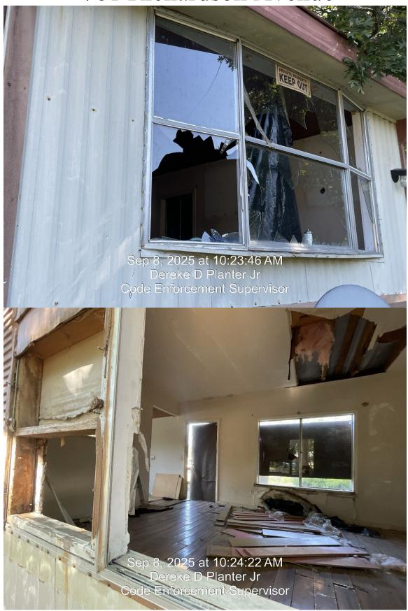
(Windows shall be reasonably weathertight with no broken glass, Interior finish shall be free of holes and excessive cracks which permit air to penetrate rooms)
