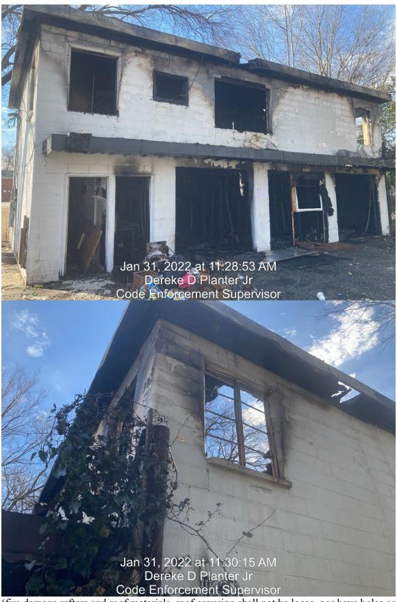
(fire damage rafters and roof materials, roof covering shall not be loose, nor have holes or leaks)
