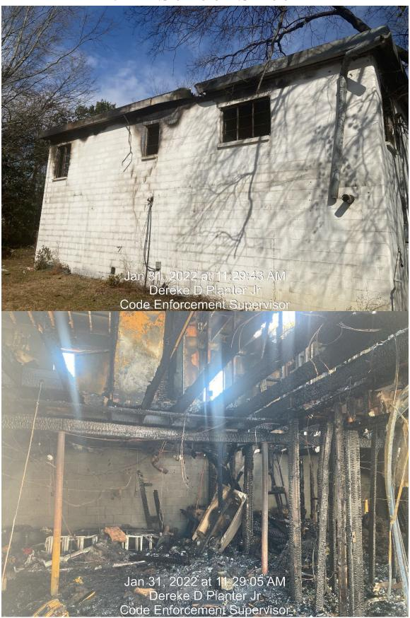
(fire damaged exterior finish not weathertight without excessive holes, cracks or rotted boards which permit air or water to penetrate rooms.)
