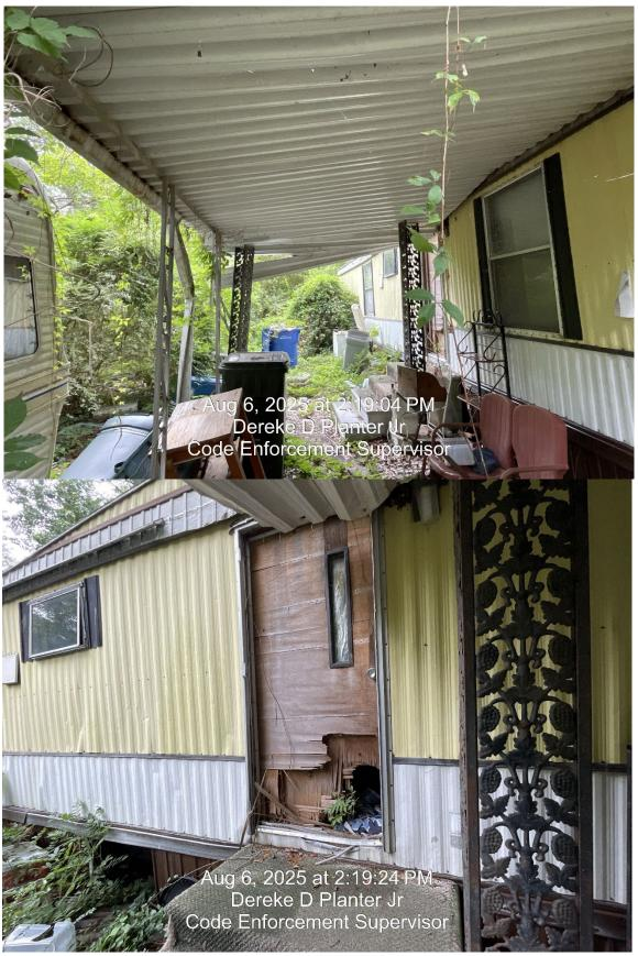
(Wall finish shall be free of holes and excessive cracks which permit air to penetrate rooms)
