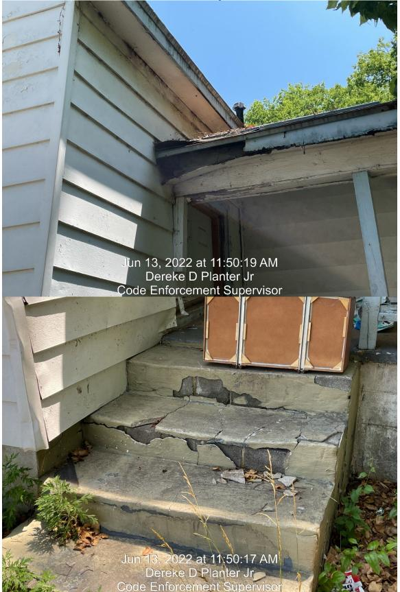
(Stairs and steps shall be free of holes, grooves and cracks large enough to constitute accident hazards; adequate posts and railings, not rotted, broken or termite damaged, shall be provided )
