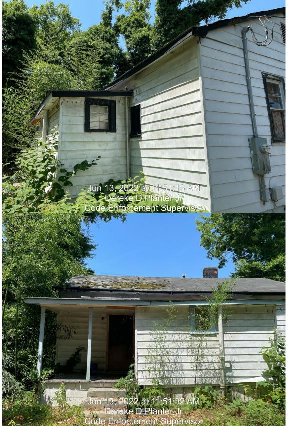
(Roof covering shall not be loose, nor have holes or leaks; Adequate posts and railings, not rotted, broken or termite damaged, shall be provided; Walls shall provide sufficient support for sheathing or exterior finish; shall provide sufficient support for sheathing or exterior finish)
