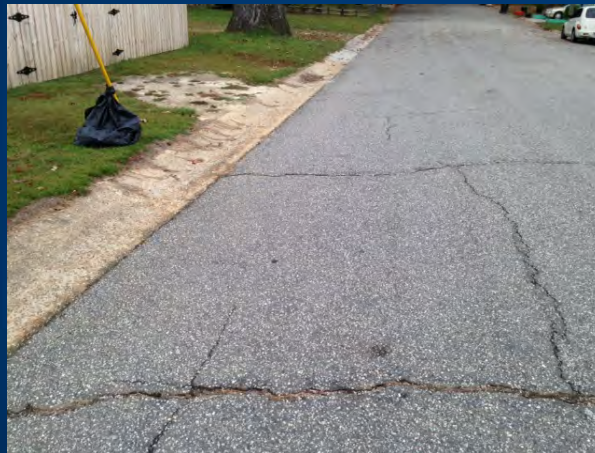
Block Cracking
