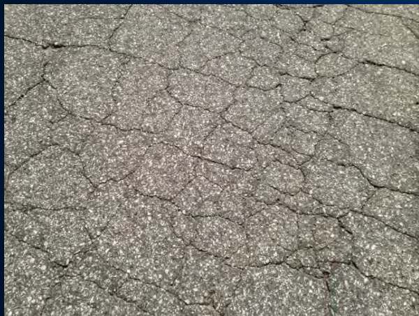
Alligator Cracking
