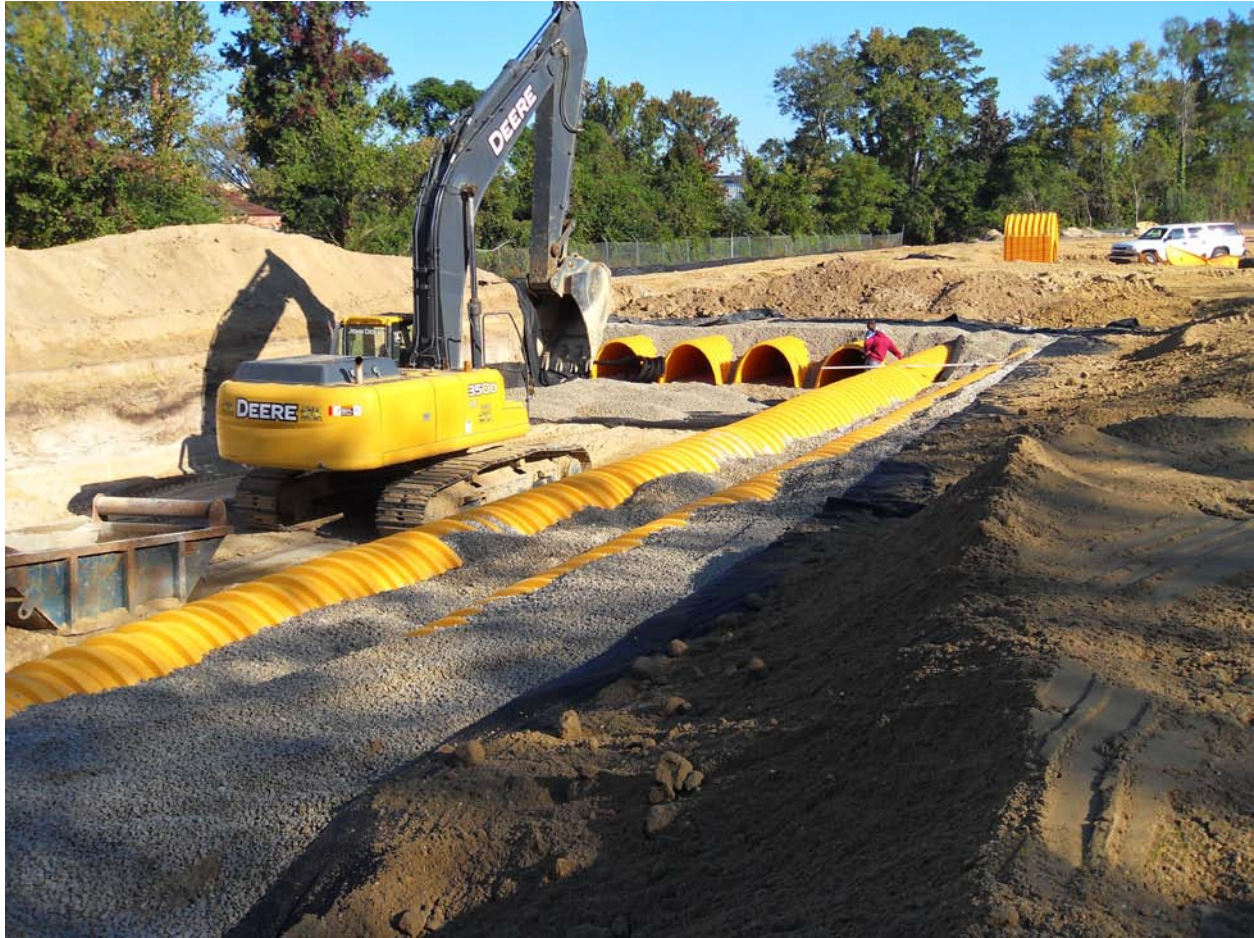
Photograph 6-1: Installation Performance Guarantees are required to ensure that BMPs such as this Infiltration Trench are installed properly
