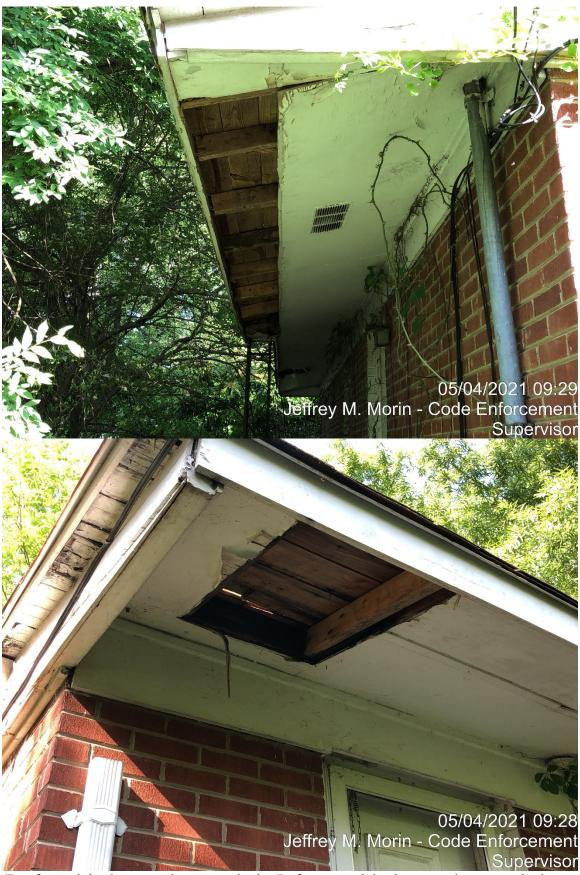
(Roof rotted, broken, sagging excessively; Rafters rotted, broken, sagging excessively or having improperly supported ends)
