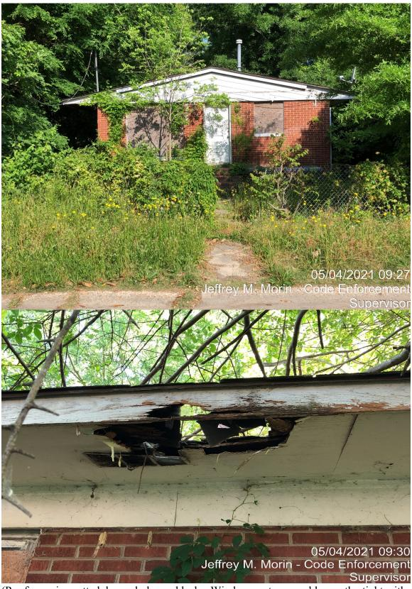
(Roof covering rotted, loose, holes and leaks; Windows not reasonably weathertight with no broken glass)
