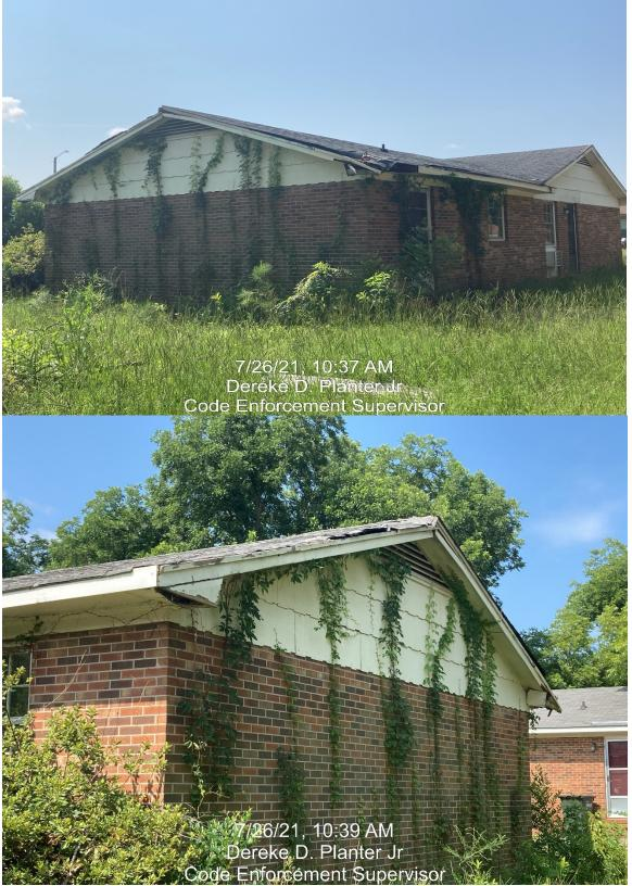
(Exterior walls cracks and rotted boards which permit air or water to penetrate rooms)
