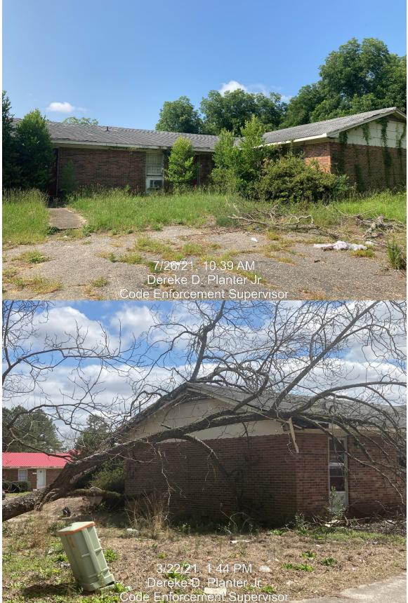
(Roof damaged from tree. Rafters shall be rotted, broken; Roof covering loose, with holes)
